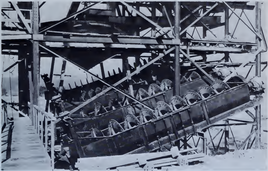
Figure 77.—Spiral classifiers for washing and dewatering sand. PX-D-32058.
